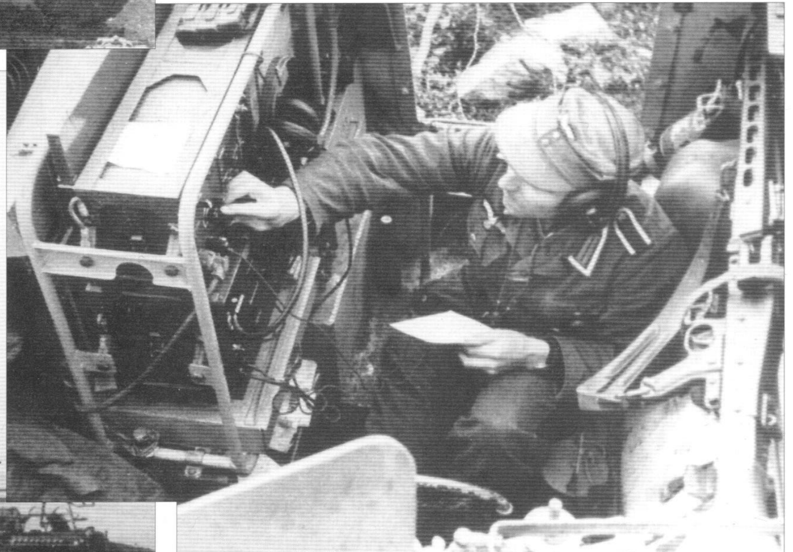
Fu 20 radio set in a Panhard scout (reconnaissance) car. The empty frames for radio sets are finely visible above. Bottom right a Sd.kfz. 223 during a German counterattack near Krivoy Rog. Eastern Front, 1943.
