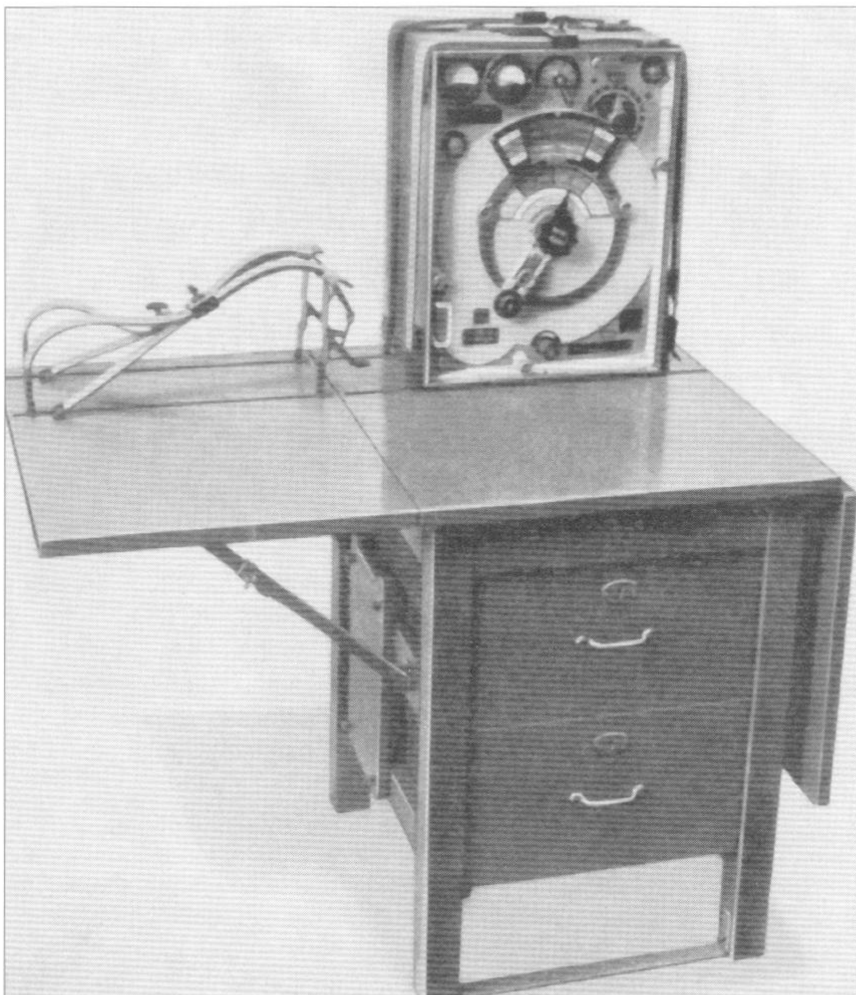
Left top a table for radios is placed. These versions still had the radios strapped to tables with webbing instead of rubber-block-mounted.
